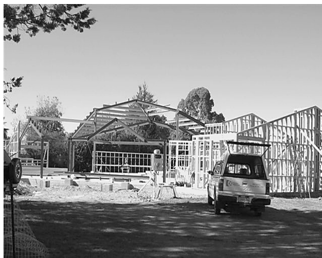
The new church building well under way
